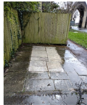
Pressure hotwash test on paving slabs.
