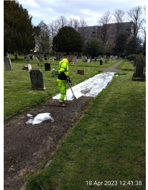
Path treatment avoiding hose getting wet.
