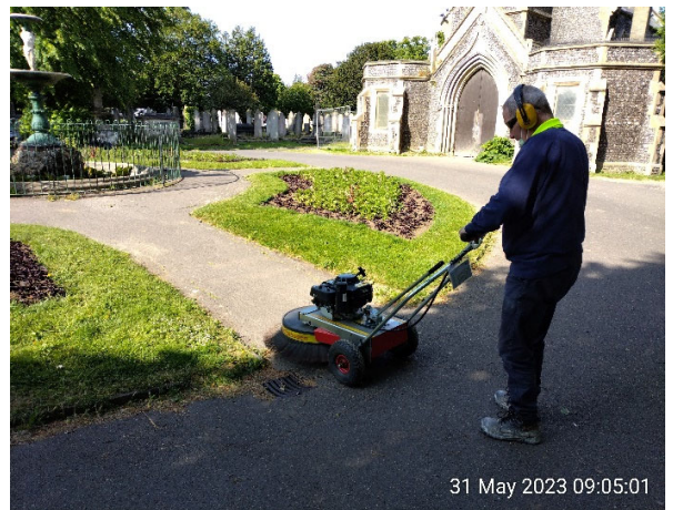
Operative using Wire weed brush.
